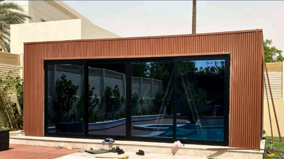
Sliding Door Installation for Enclosed Majlis – Private Villa, Dubai
