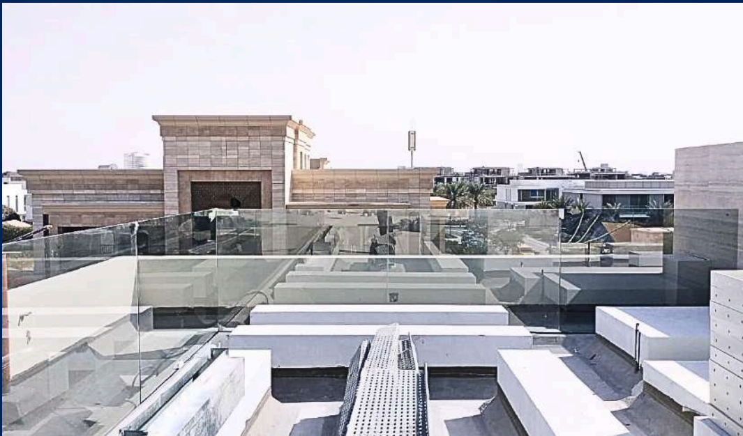
Clear View Handrail Installation – Model Consultants (B2B), Nad Al Sheba, Dubai
