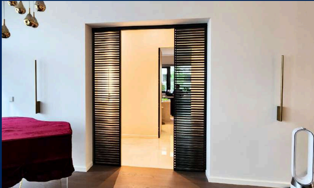
Installation of Slim Sliding Door – Private Client, Dubai
