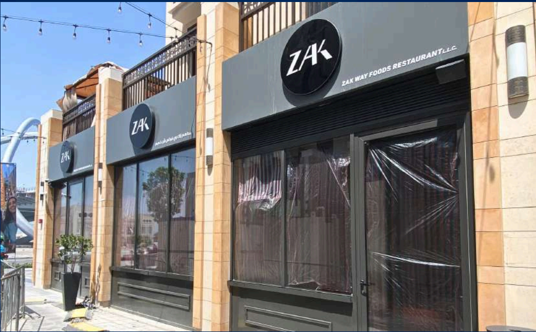
Exterior Glass Wall Installation – ZAK Restaurant, Dubai
