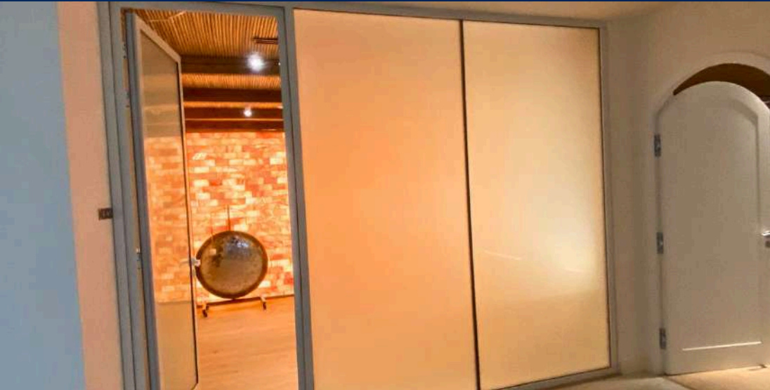
Smart Glass Installation – Model Consultants (B2B), Dubai
